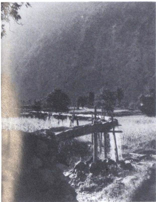
3. Wooden aqueduct for irrigation water
